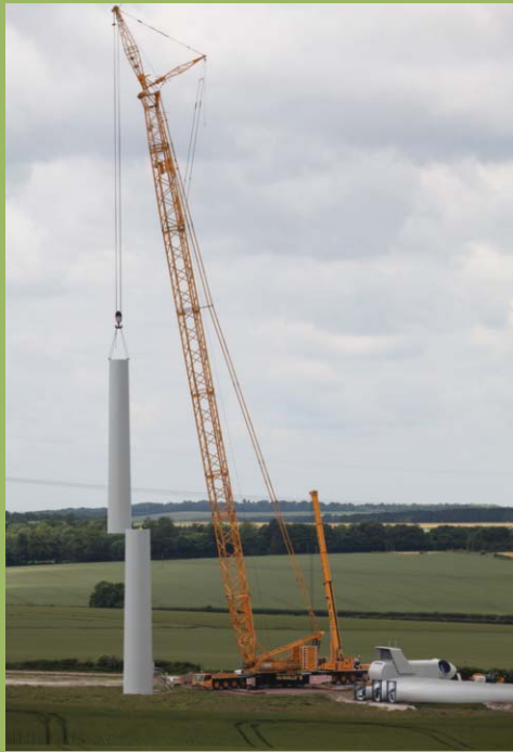
1. The tower sections are connected together.
