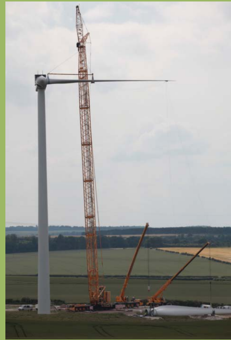
3. The blades are fixed in place.
